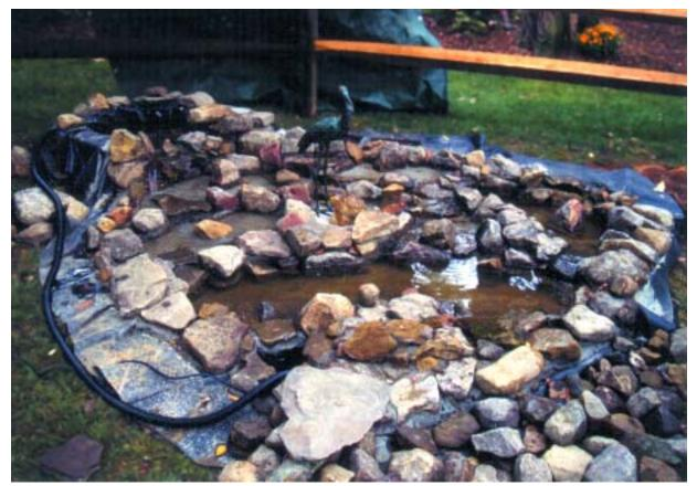
The plumbing from the submersible pump in the hidden reservoir would be buried to the entry point at the top of bird pond.
