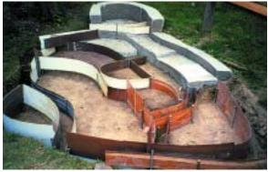
Flexible and thin wall panels were used to create forms for the concrete base
