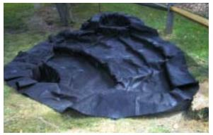
A geotextile fabric protects the liner for the long life of the pond construction.
